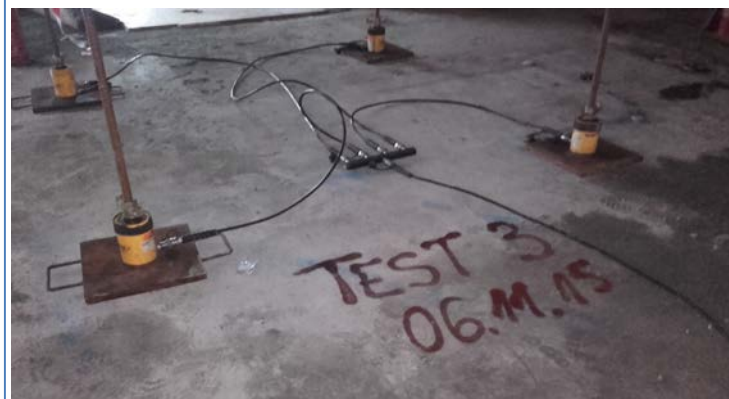
Test area in no.6 Stanhope Gate building
